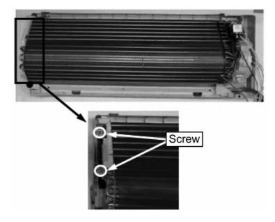
8 Loosen the fixing screw (1 screw) which fixes the cross flow fan to the indoor motor.
